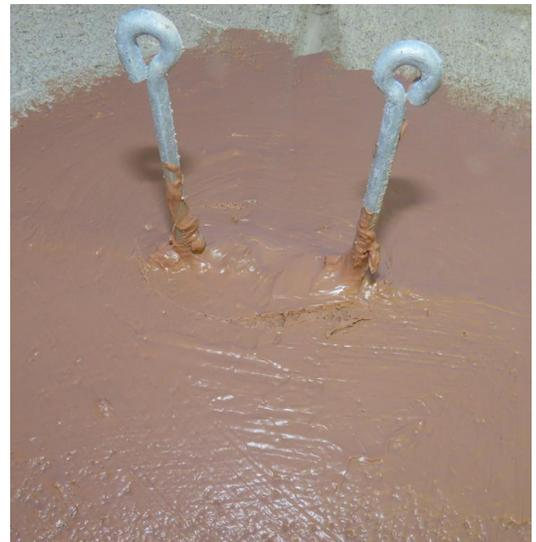
***We recently started pre-coating the masonry pintles, taking the time to detail each penetration ahead of the spray or roll installation. We immediately saw a substantial benefit to the installation with less failure and rework.***
